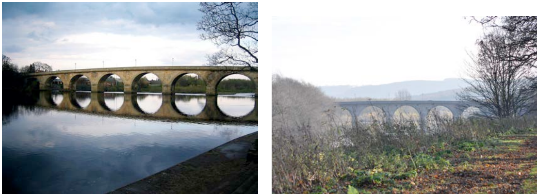
Views of Hexham Bridge
